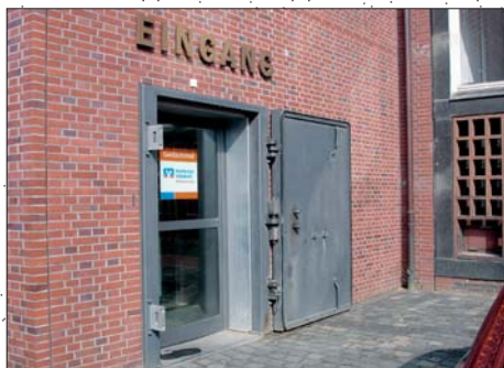
Hub-Schwenk-Türe (HST), schwellenfrei.
