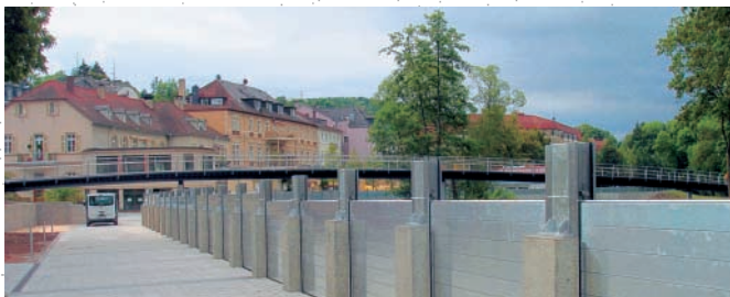
View from the foyer to the Luitpoldsteg
