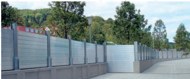
Rose Garden behind the demountable flood defence barrier
