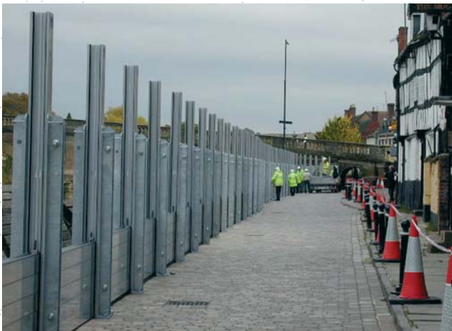
Full system erection at minimum defence height
