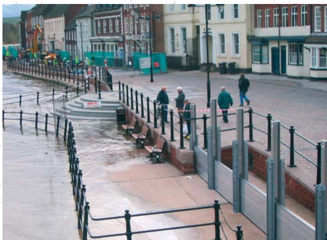
Firstly, full height barrier system installed
