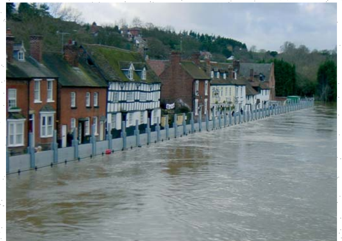
Holding back rising flood waters
