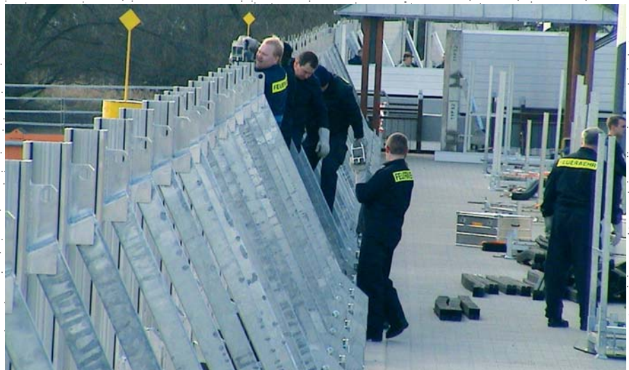
Assembly of the IBS systems by the Civil Emergency Services
