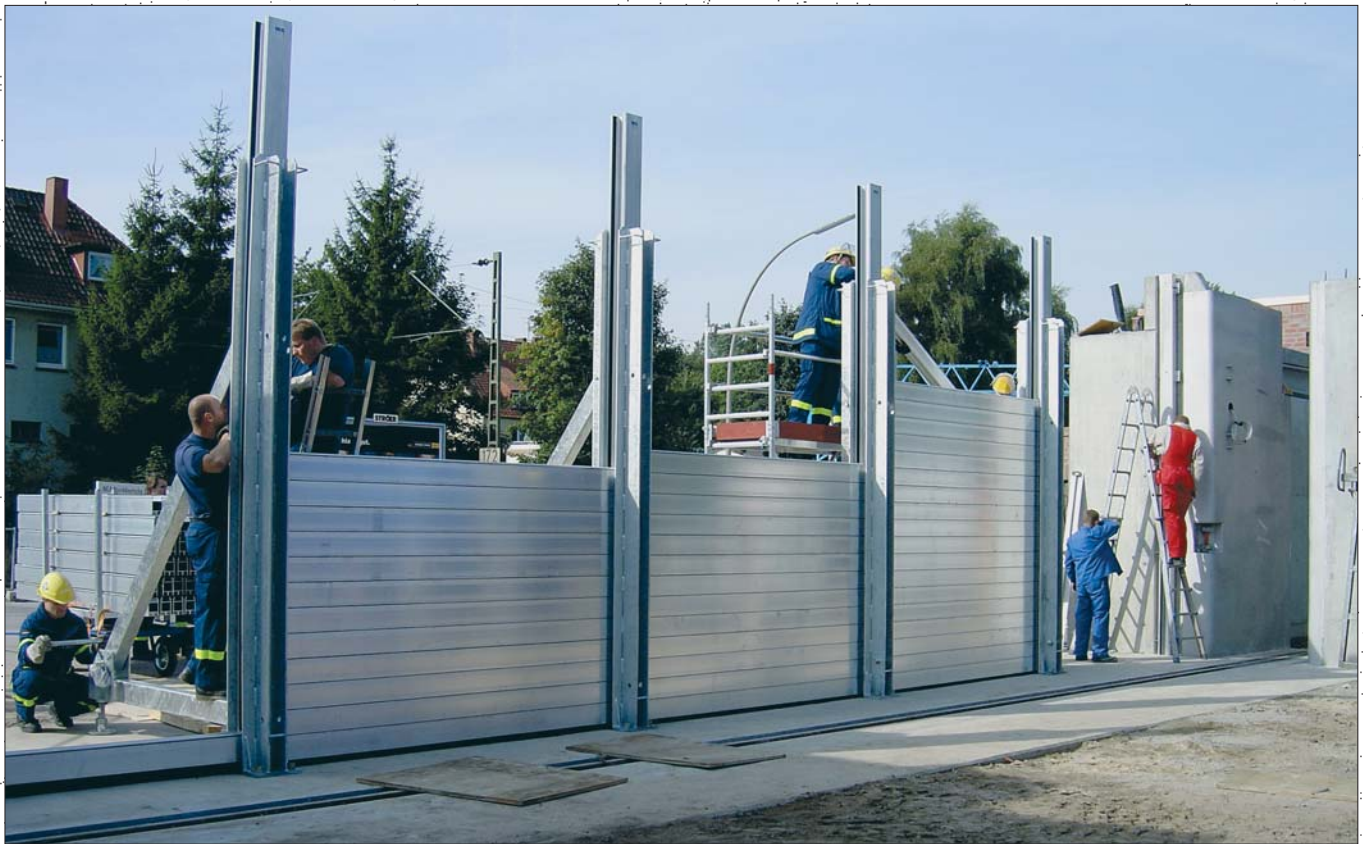
Trial set-up of IBS demountable flood defence systems in Hamburg
