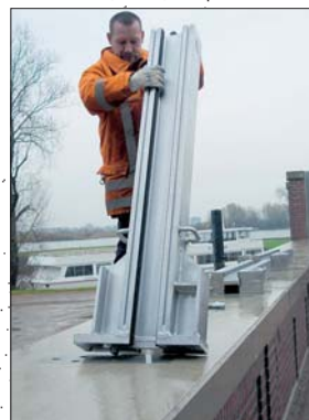
Exact fitting of the post through locking
