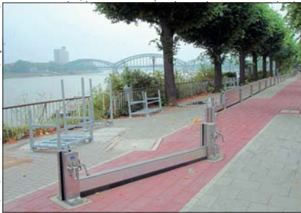
Corner support posts
