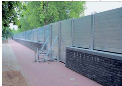
Transit area with height transition
