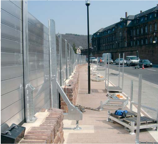
Simple to erect – the IBS demountable flood defence system
