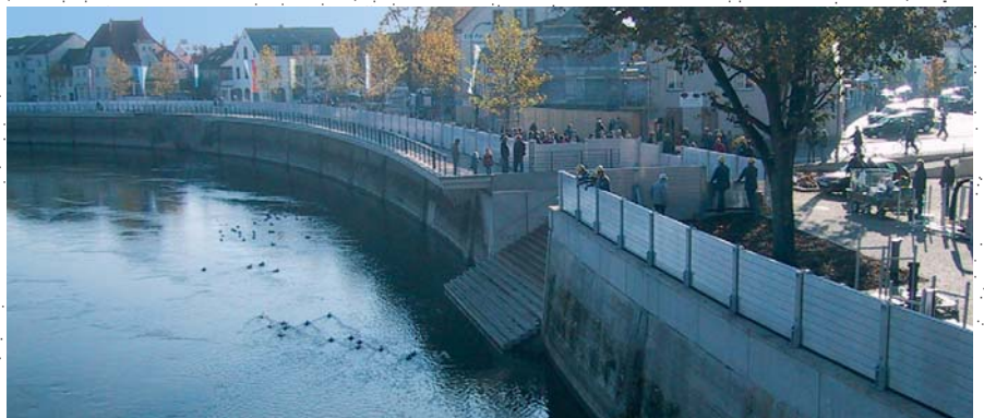
The demountable flood defence system along the River Danube
