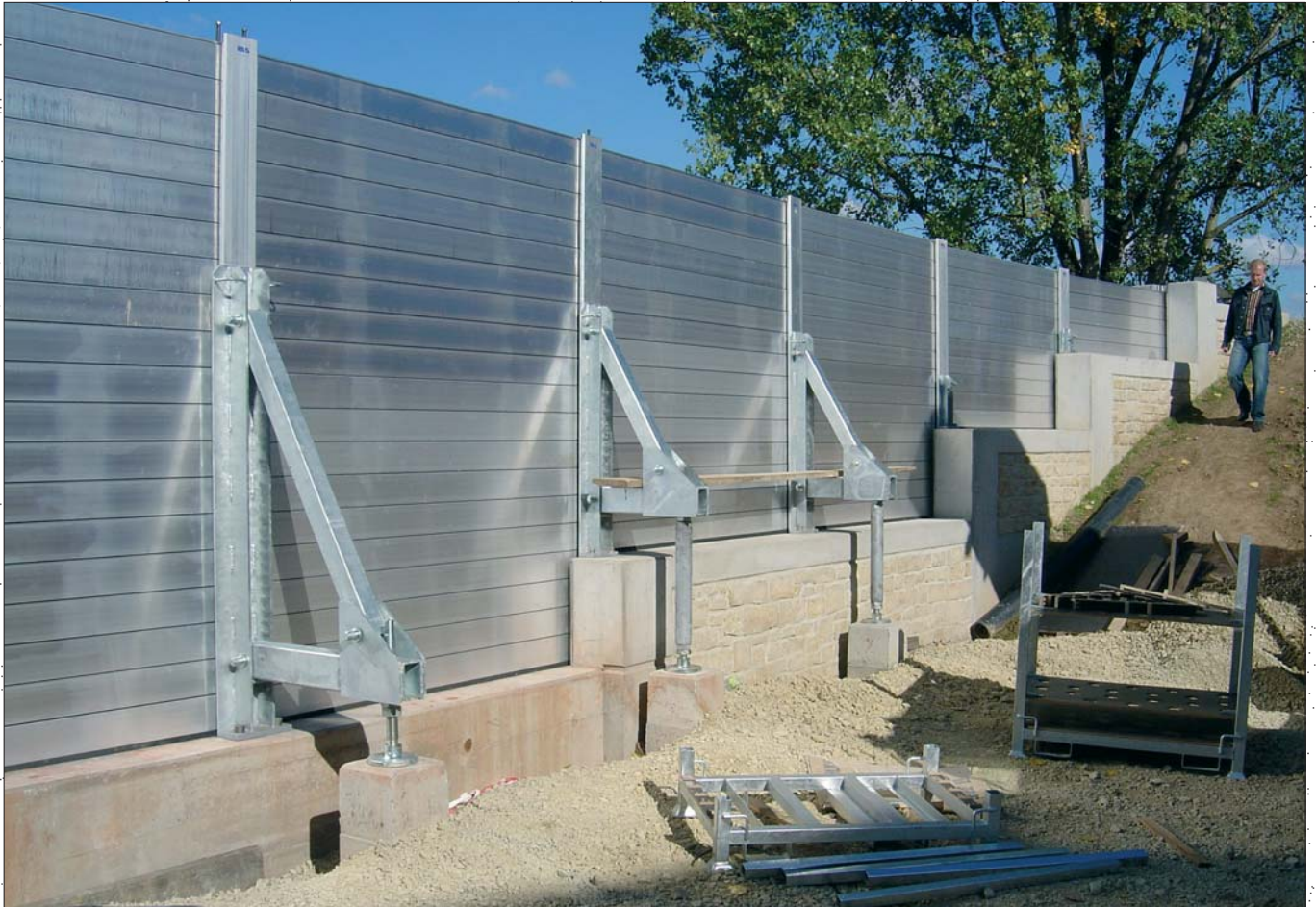
Foundations with varying levels are no problem for the demountable flood defence system.
